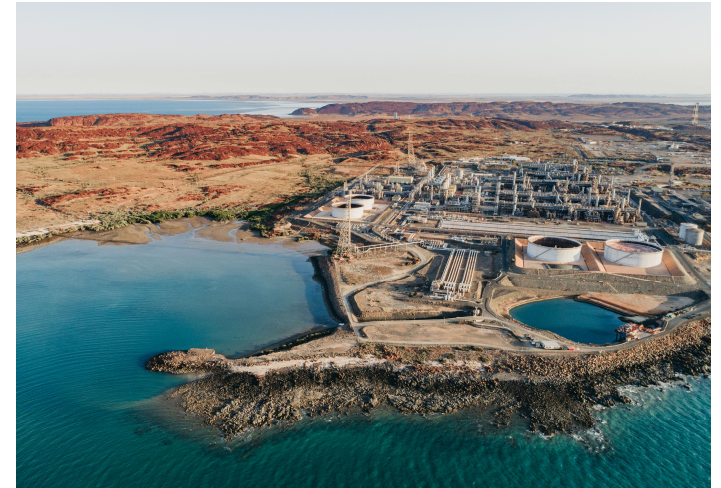
The Woodside-operated Karratha Gas Plant in Western Australia.
